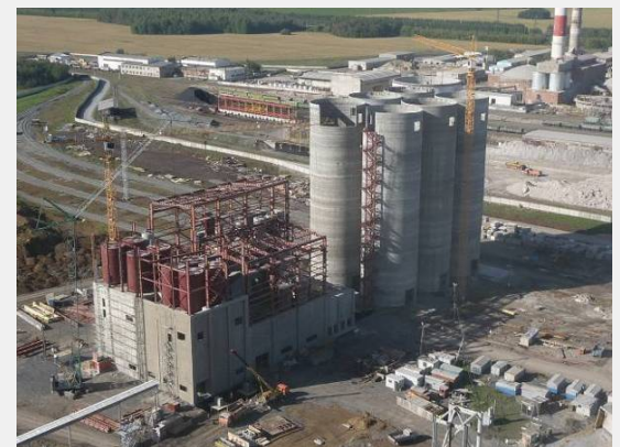
Cement mill and delivery station
