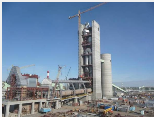
Tower and kiln basement
