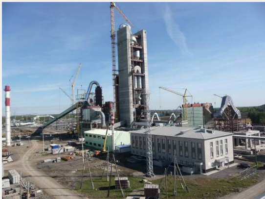
Overview of new line
